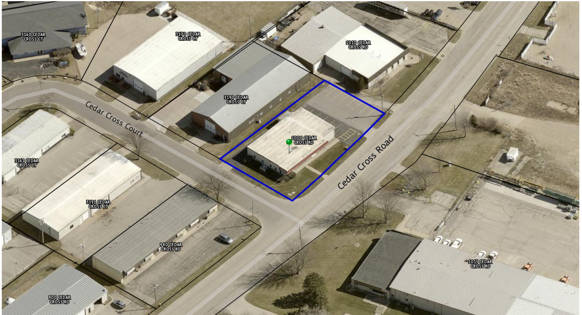
Oblique view of subject property from west, March 2024 imagery
