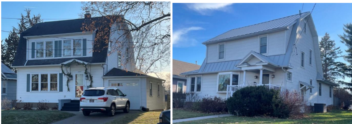
2425 Asbury (left) and 2545 Asbury (right) (Colonial Revival: Dutch Colonial)
