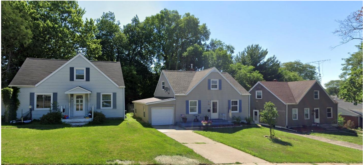
2154, 2144, and 2130 Morningview, constructed by Vernon Carris c. 1948-1949. Source: Google, photographed July 2022
