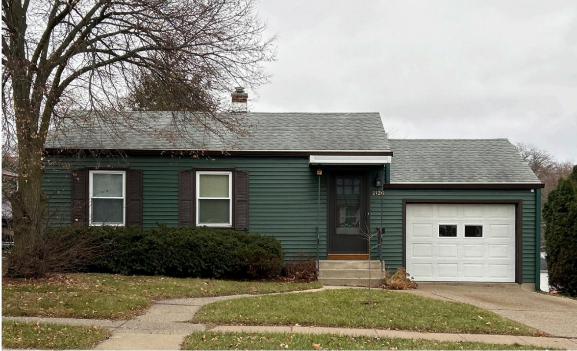
2126 Broadlawn, constructed by Vernon Carris c. 1948-1949.
