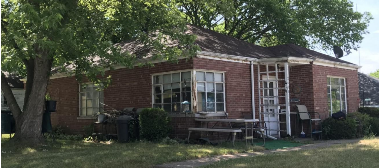
2098 Morningview, a typical Type 3 Deereville house, which notably retains the original steel windows that were used in all of the Deereville houses
