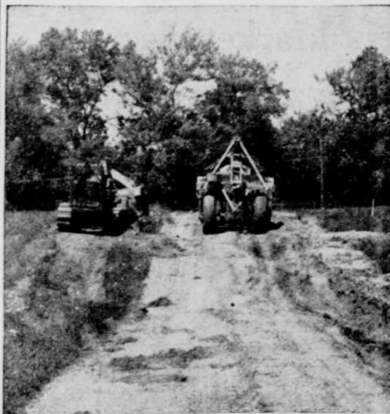
Street grading equipment pictured above has rolled into action and work has started to round into travel shape nine streets in the newly annexed lands at the west corporate limits of Dubuque. There are slightly more than 59 acres of land in the annexed territory and streets to come under the grading project include Hillcrest, Avalon, Broadlawn, Morningview, Chaney, Ogilby, Mullin, Valleyview, and Asbury road. Contract for the grading project recently had been let by the Dubuque city council to Sumner Sollitt and company, of Chicago. (Telegraph-Herald Photo)
