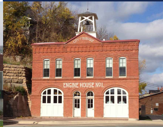
Old Engine House #1 | 1805 Central Ave. Economic Mobility and Neighborhood Support
