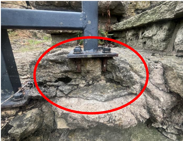
Figure 454. Spall at the end of a stone stair tread at the east stair.
