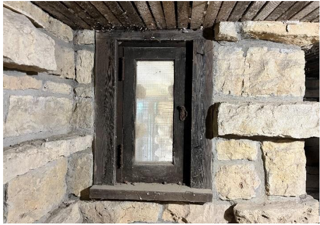
Figure 94. Window opening at sides of stone pier, operable from the interior.
