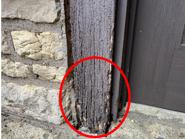
Figure 515. Distress at bottom of vertically oriented wood member.
