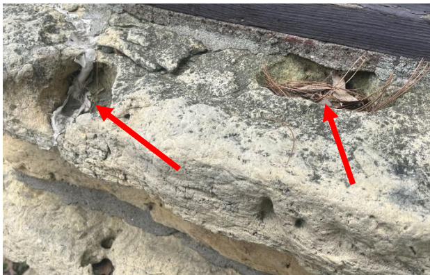
Figure 190. Deep pockets and pits in the stone.
