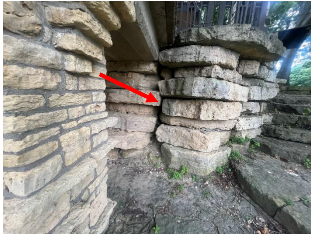
Figure 480. Crack aligned with the edge of the covered stone terrace deck slab.
