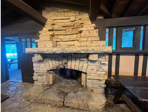
Figure 422. Arched firebox opening and hearth stone at interior fireplace.
