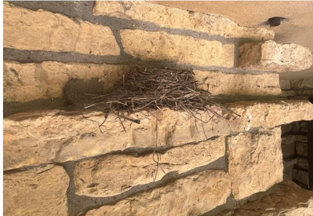
Figure 193. A bird nest adjacent to projecting stone units.
