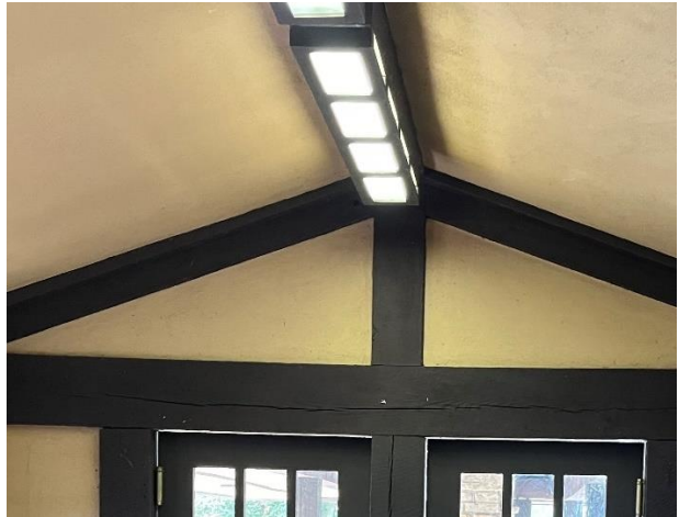
Figure 446. Non-original light box mounted to the ceiling of the north annex.
