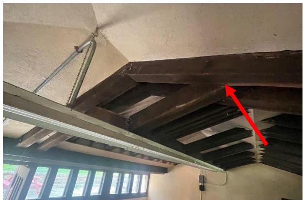
Figure 234. Wood roof framing at dormers.
