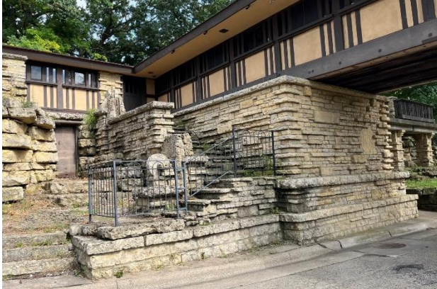
Figure 387. Overview of east stair.
