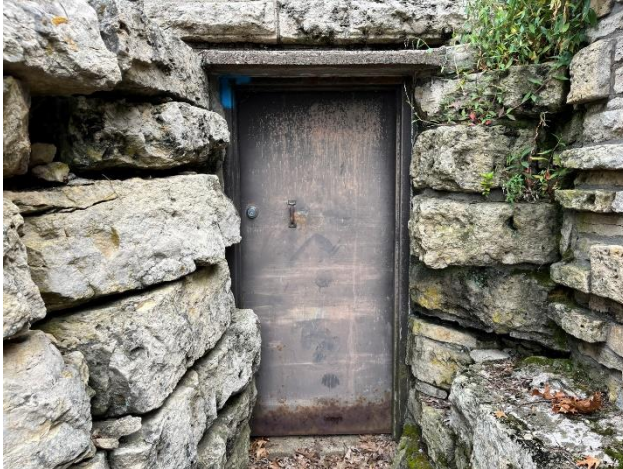
Figure 349. Non-original steel-framed door.
