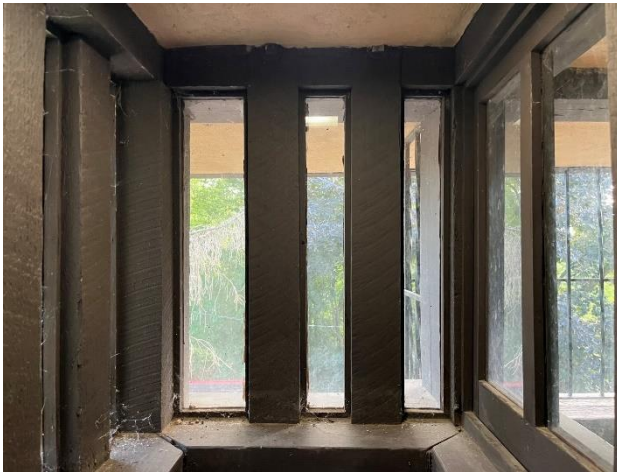
Figure 338. Fixed sash window near balcony.
