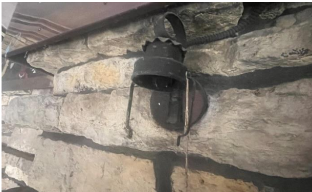
Figure 169. Surface-mounted lantern, with the lamp of the light fixture missing.
