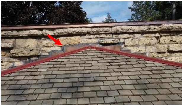
Figure 110. Copper flashing at stone chimney.
