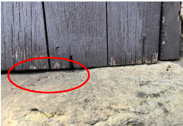
Figure 217. Minor wood deterioration at doors including chips and splits along the base of door leaves.
