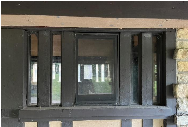
Figure 336. Exterior view of single sash casement window.
