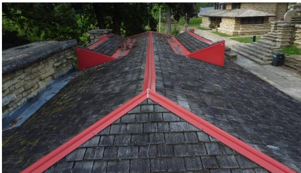
Figure 259. Overview of hip roof.
