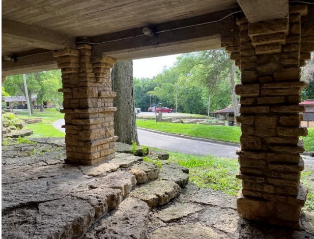
Figure 364. Stone piers with haunches support the concrete slab.
