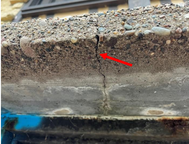
Figure 516. Cracking at concrete lintel with evidence of moisture staining and infiltration along the crack.
