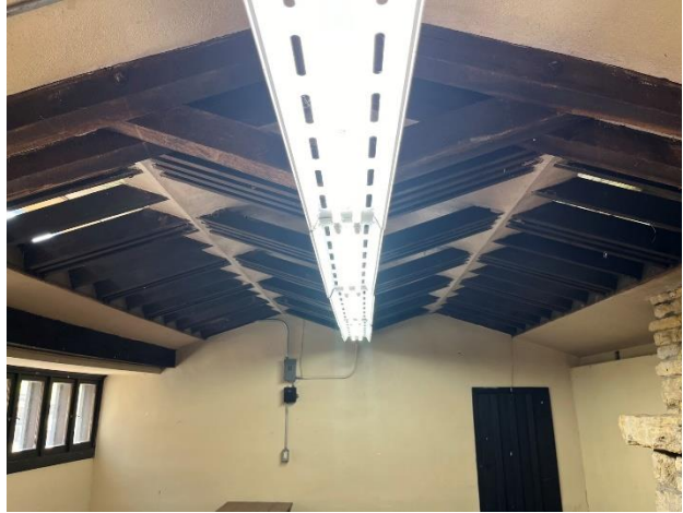
Figure 230. The interior finishes partially concealing the roof framing.
