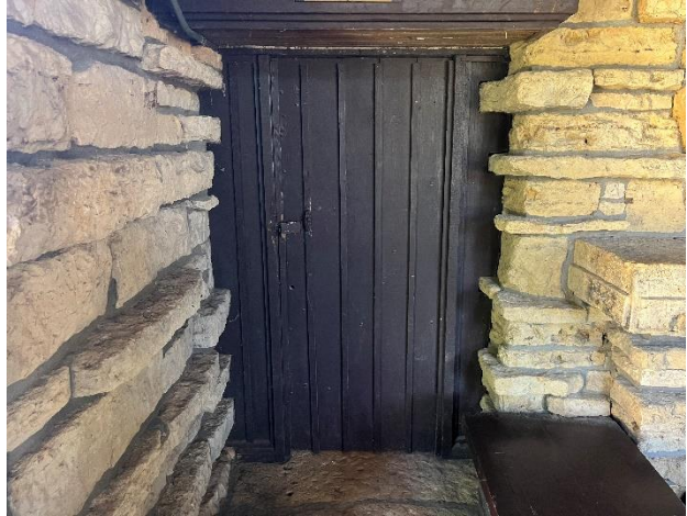
Figure 140. Vertical reinforcing on the main gathering room face of the door.
