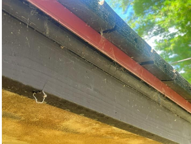
Figure 113. Wood fascia with coved wood trim located below the drip edge flashing.
