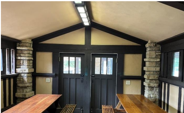
Figure 412. Plaster ceiling at the north annex.
