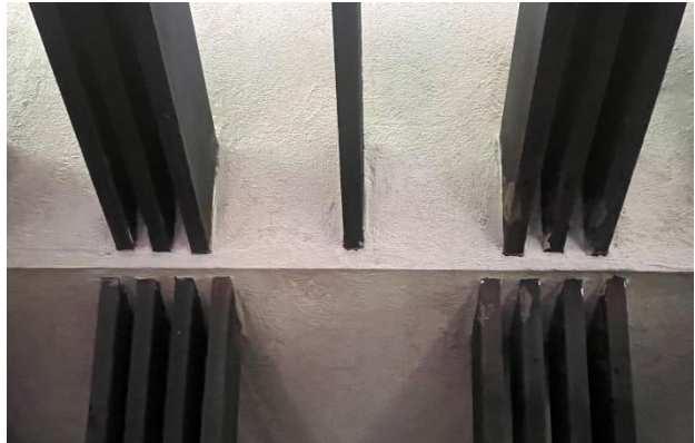
Figure 232. Four diagonal bracing members offset in their alignment with the three rafters so that they fit within the space between.
