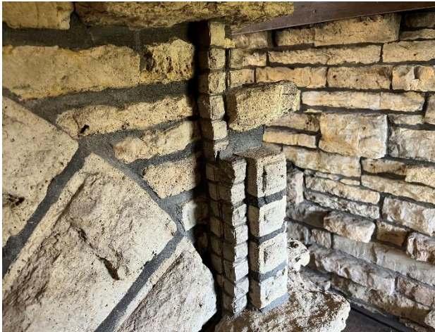
Figure 154. Small and large stacked square stone units.
