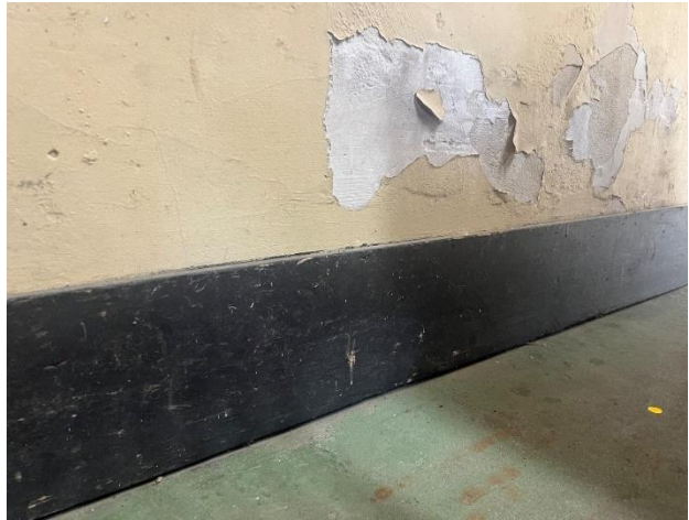
Figure 272. Wood baseboard without projecting wood trim above.
