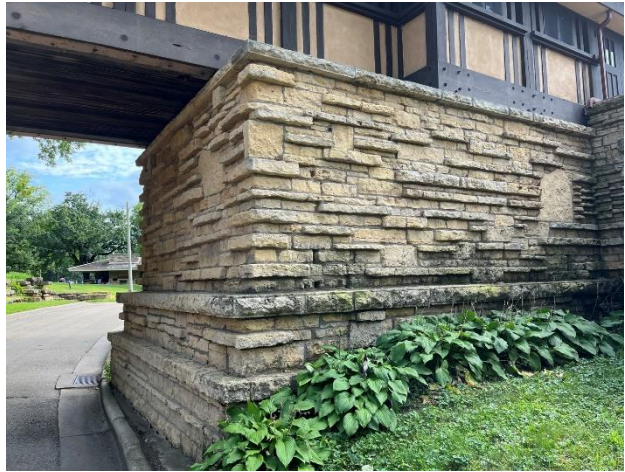
Figure 301. The reservoir forms a raised base for the one-story building with lookout tower.
