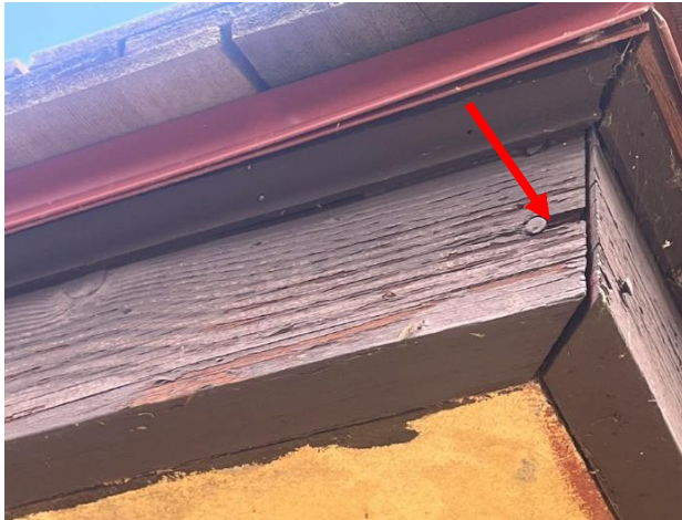
Figure 200. Minor checks and splits at the ends of some wood fascia boards.
