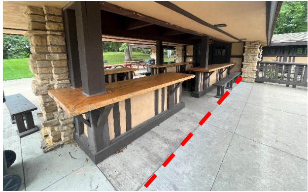
Figure 376. Concrete floors at the covered patio and north terrace. Note that the concrete at the covered patio is different than the concrete at the north terrace.
