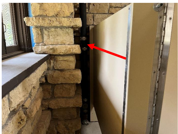
Figure 181. Vent pipe at the restroom extends through the floor slab and through the roof framing.
