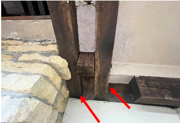
Figure 235. Ends of wood framing members for dormer roof.
