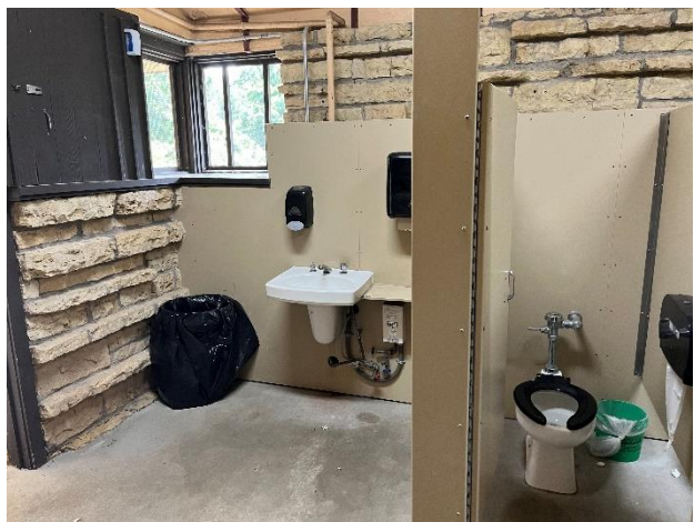
Figure 179. Typical bathroom fixtures and wood-framed partition wall installed as part of the 2005 restroom renovation.
