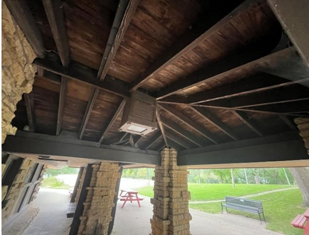
Figure 322. Roof framing at east entrance vestibule roofs.
