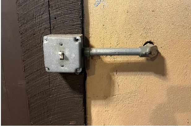
Figure 437. Non-original surface-mounted conduit and light switch.
