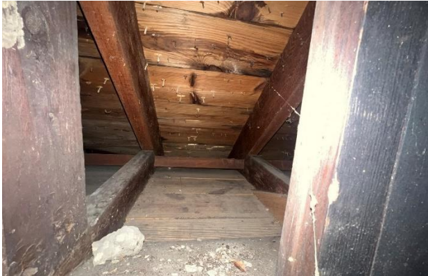
Figure 231. Eave framing at wood roof soffit.
