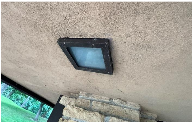
Figure 443. Recessed lighting at stucco soffit is of similar design as the interior recessed lighting.
