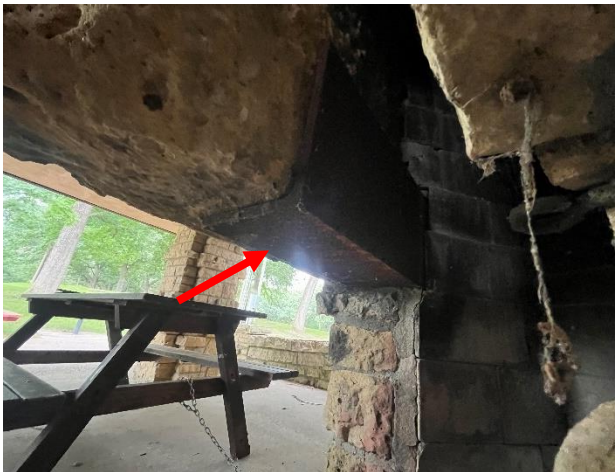
Figure 420. A 6x8 steel channel supporting stone unit above,
