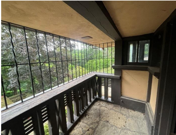
Figure 358. View of the balcony stone-paved deck.
