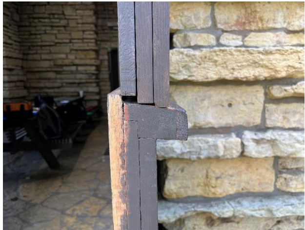
Figure 99. The doors consist of three plies of 1x board and measure approximately 2-3/8 inches thick.
