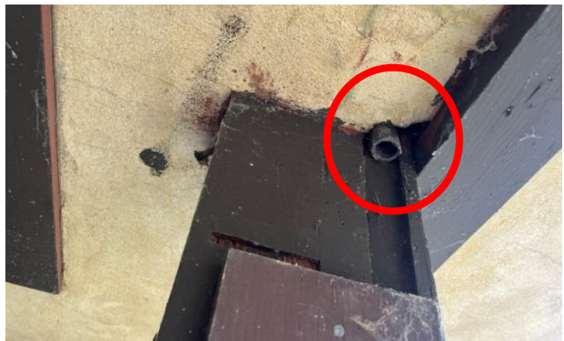
Figure 170. Abandoned conduit and routed wood channel at recessed vestibule.
