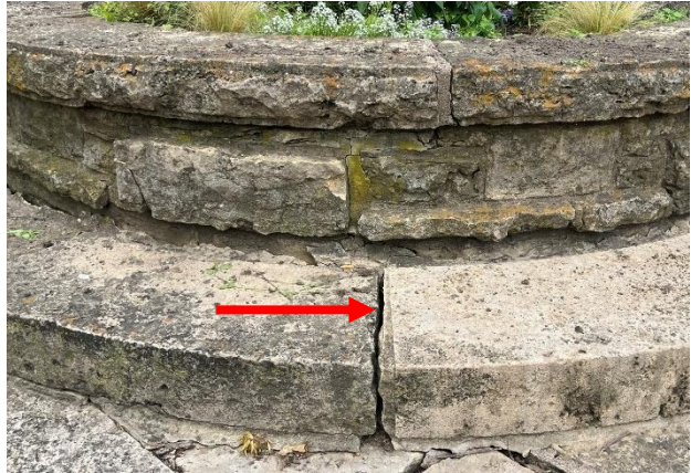
Figure 69. Open mortar joints at circular planter at Veranda Rooms terrace.
