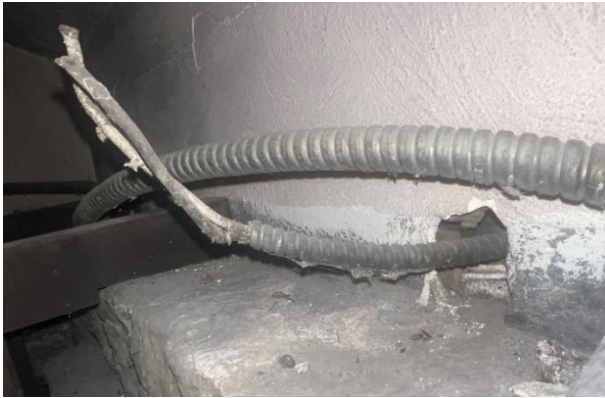
Figure 165. Coiled flexible metal conduit.
