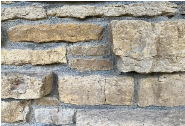
Figure 237. Typical stone units at wall.
