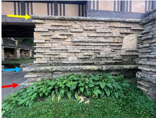
Figure 320. Typical wall area showing lower watertable (red arrow), upper watertable (blue arrow) coping band (yellow arrow).
