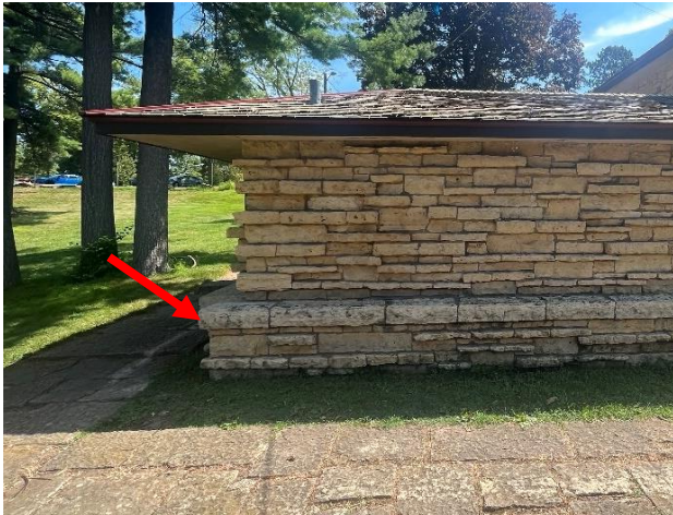
Figure 79. Stone watertable at base of building elevation.
