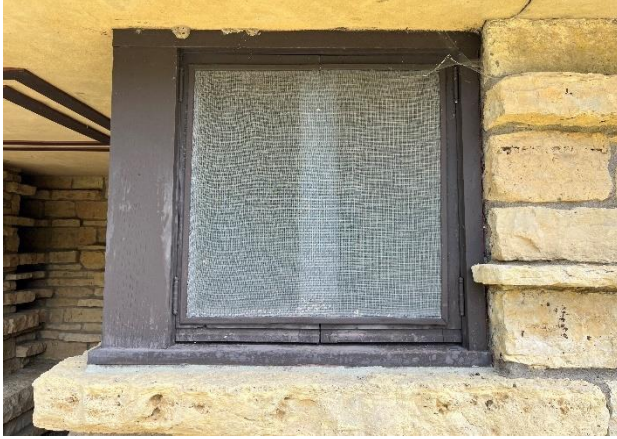
Figure 93. Wood-framed screen mounted over the exterior of the sash, making the windows inoperable.
