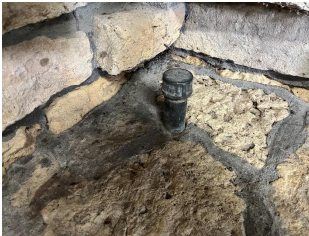
Figure 176. Capped pipe set in floor of community room likely supported a radiant heating system that has since been removed.
