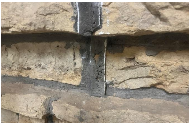
Figure 132. Evidence of previously existing interior partition wall.
