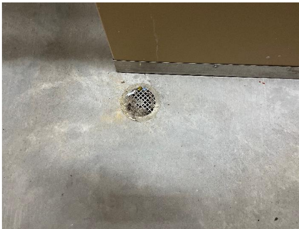
Figure 180. Floor drain at the restroom.
