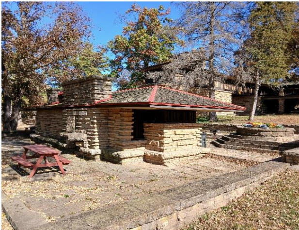
Figure 37. Pavement surrounding Veranda Rooms.
