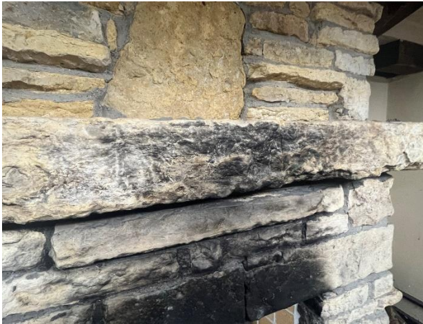
Figure 303. Dark soiling, likely soot, above the north fireplace.
