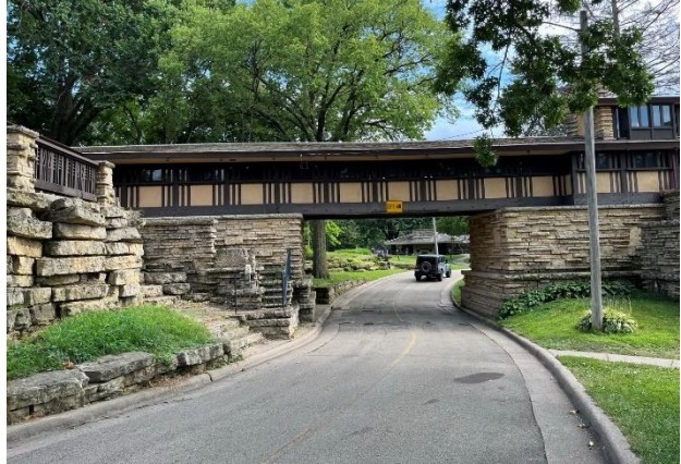
Figure 307. View of the bridge from the north.
