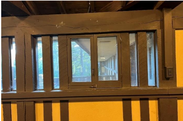
Figure 330. Interior view of casement sash with fixed sidelights.
