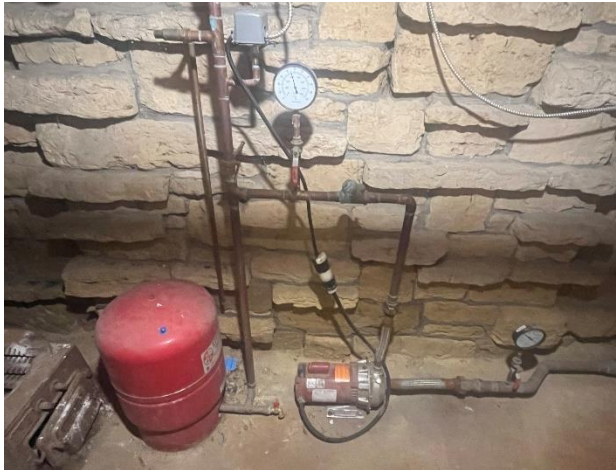
Figure 178. View of water heater, booster pump, and copper piping installed as part of the 2005 restroom renovation.
