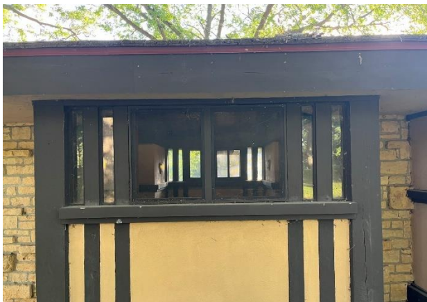
Figure 334. Exterior view of two-light casement windows
