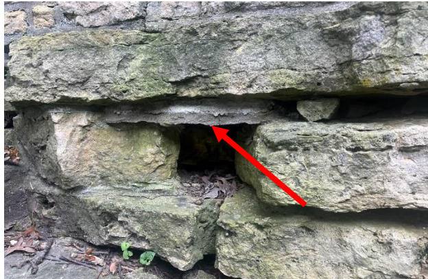
Figure 451. Spalling and erosion of stone along a mortar joint. Arrow shows continuous mortar above a stone spall.
