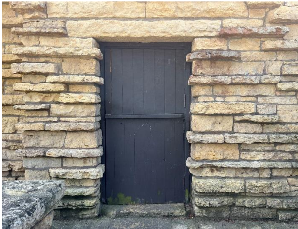
Figure 98. Dutch door with a stone lintel.
