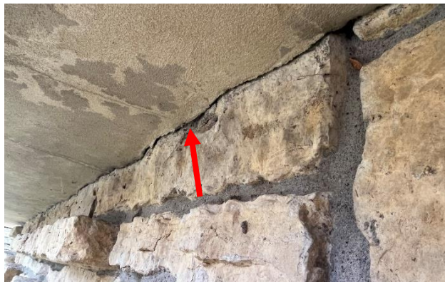
Figure 191. Continuous gap, measuring 1/8 inch wide, between the materials.
