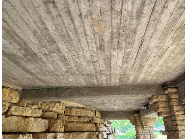
Figure 365. Concrete deck with slab with formboards.
