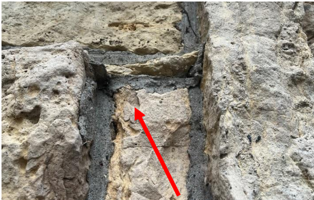
Figure 478. Chipped stone ledge unit.
