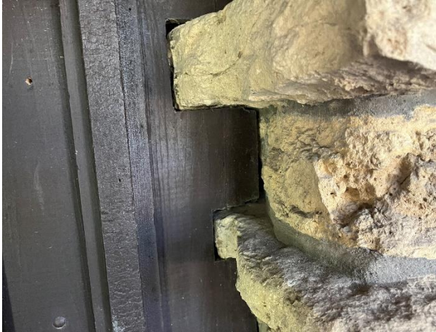
Figure 139. Wood panel transom notched around the profile of the stone.
