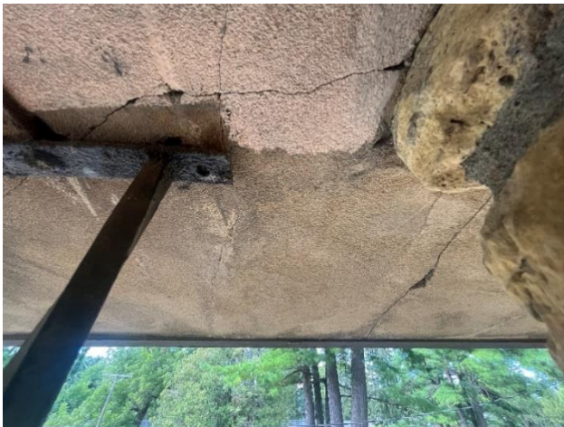
Figure 210. Cracks extending from anchor locations for the wrought iron grille.
