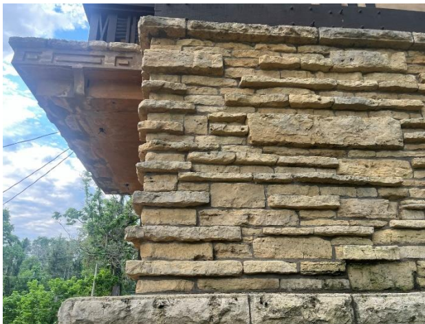
Figure 317. Typical stone cladding at Bridge Complex.
