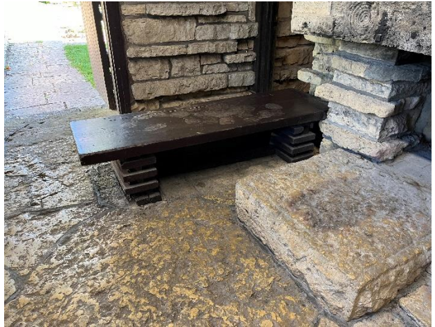
Figure 160. The front edge of the bench aligned with the outside of the mantel support stones.
