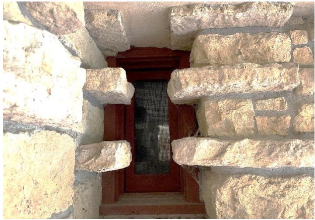
Figure 96. Metal mesh screening stapled to the exterior face of the sash.
