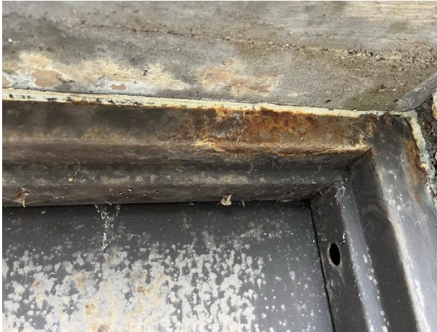
Figure 518. Corrosion at the head of the door frame.
