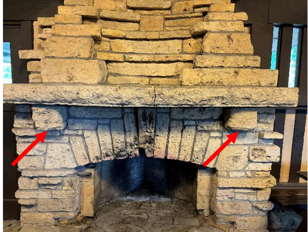
Figure 423. Horizontal tooled mantel supported by two stone blocks.
