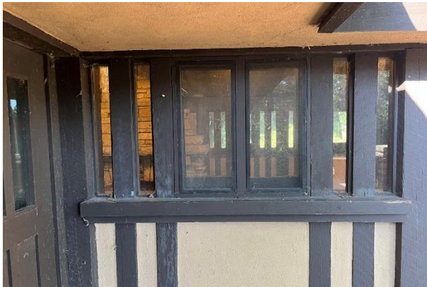
Figure 332. Exterior view of casement sash with fixed sidelights.
