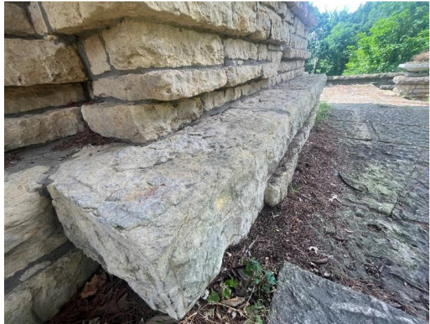
Figure 80. Rock-faced finish stone watertable unit.
