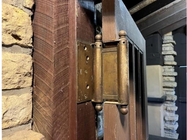
Figure 415. Original double-action hinge at door.
