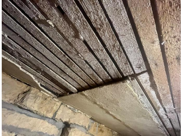
Figure 136. The ceiling in the mechanical room is plaster on wood lath.
