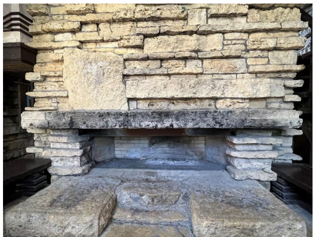
Figure 147. Stone mantel spanning across the firebox opening.
