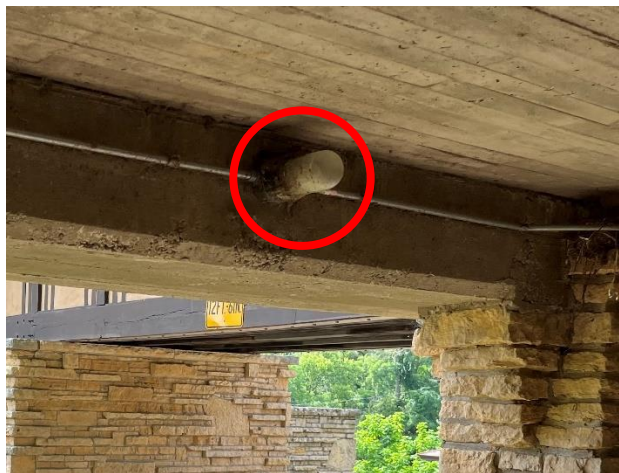
Figure 448. Non-original surface-mounted light at stone terrace.
