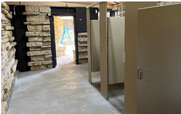
Figure 125. Polished concrete flooring in restrooms.
