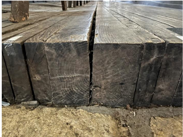
Figure 498. Open joint between wood floor beams resulting from warping.
