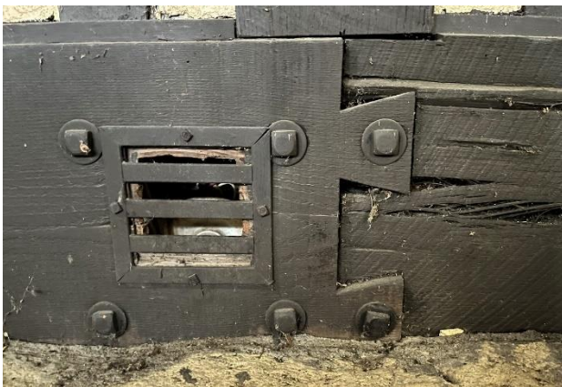
Figure 407. Dovetail connection between framing members.
