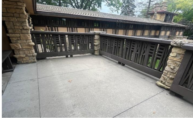
Figure 373. Concrete paving at the north terrace.
