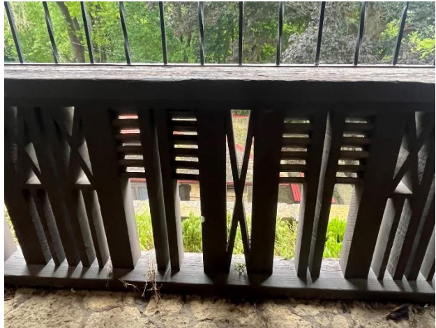
Figure 359. Original wood railing sitting on stone pavers.
