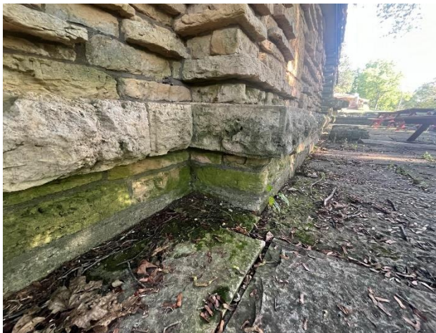
Figure 239. Projecting lower watertable.
