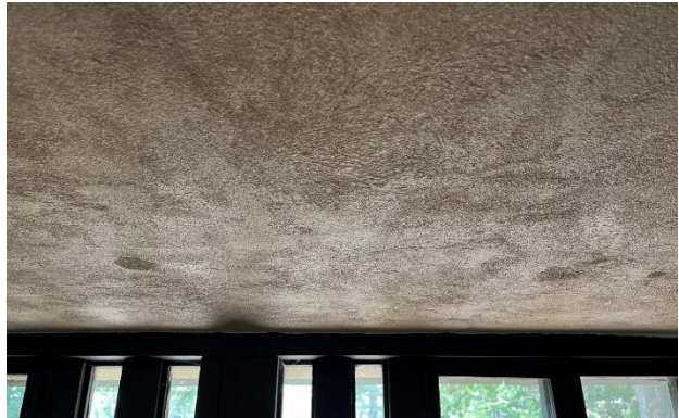
Figure 413. Plaster ceiling at the west room.
