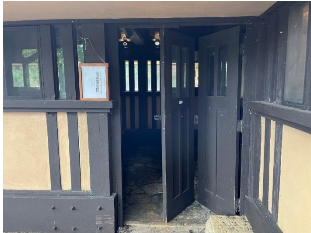
Figure 348. Exterior view of bi-fold door in partially folded position.
