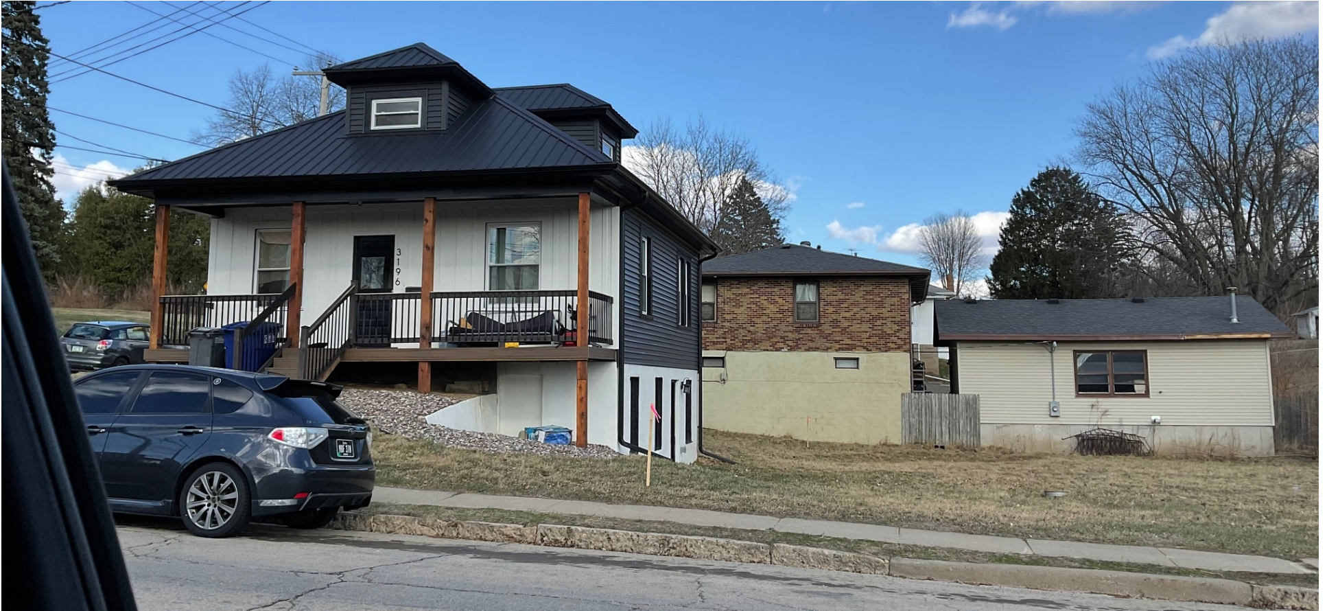
Photos of subject property, March 25, 2025
