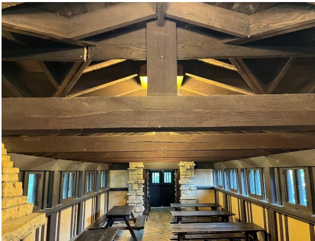
Figure 324. Roof framing at east room.
