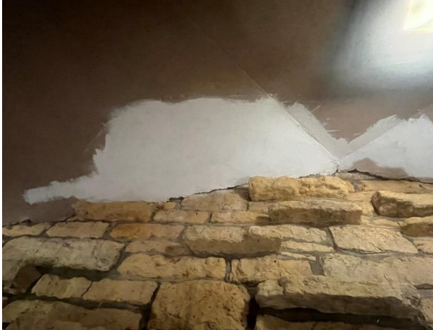
Figure 135. Previous plaster patches at the sides of the chimney.
