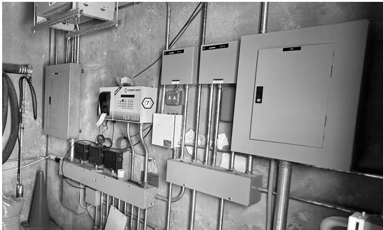
ER FUEL DISPENSION PANEL AND ASSOCIATED POWER SUPPLY IN PUMP HOUSE
