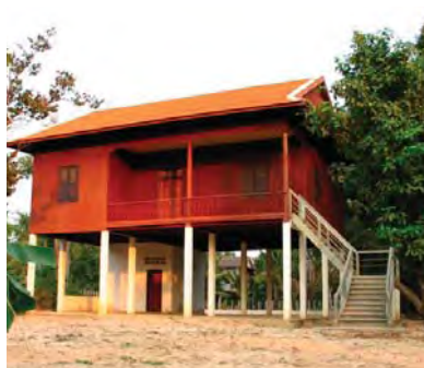
2. Raised Above Flood Plain
