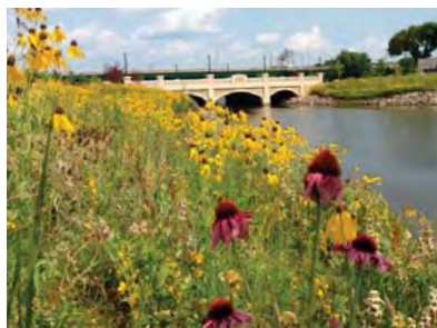
Bee Branch Creek Restoration
